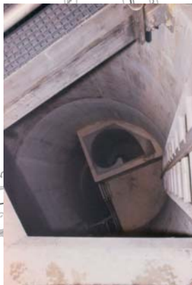
Typical Vortex Drop Structure (Viewed from above)
