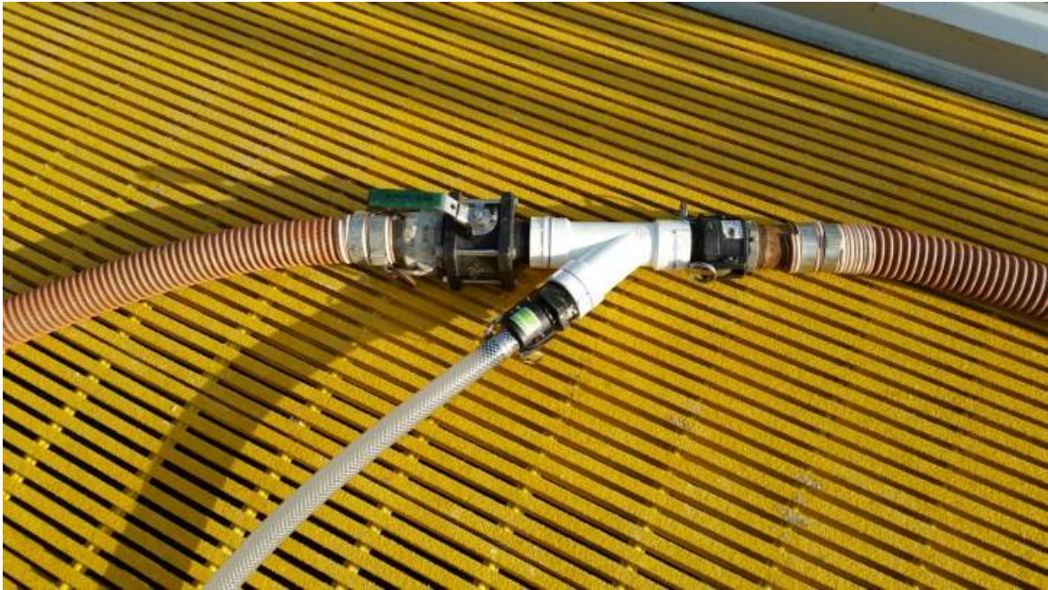
Figure 2.2 PVC Splitter and Valve
