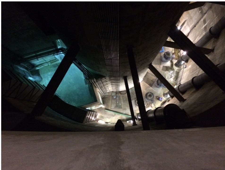
Figure 4-4. Wet well/dry well pump station - one circular shaft with wet wells and pumps on perimeter
