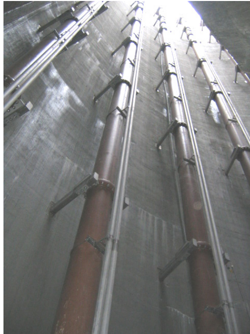
Figure 2-6(B). Pump guide bars
