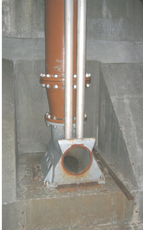
Figure 2-8. Conceptual pump discharge connection
