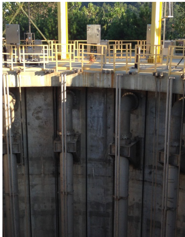
Figure 2-5(A). Pump guide bars
