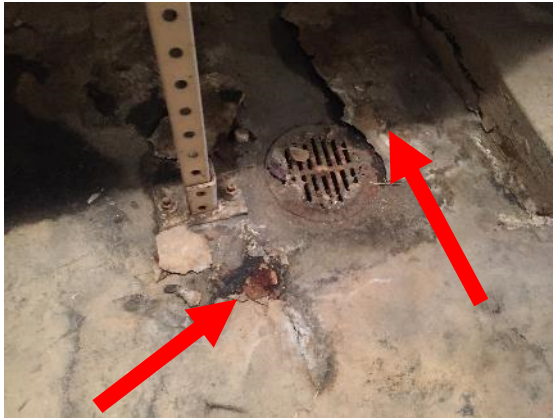
Figure 4-2 Concrete at the Blower Room Floor Drain Above Wet Well B
