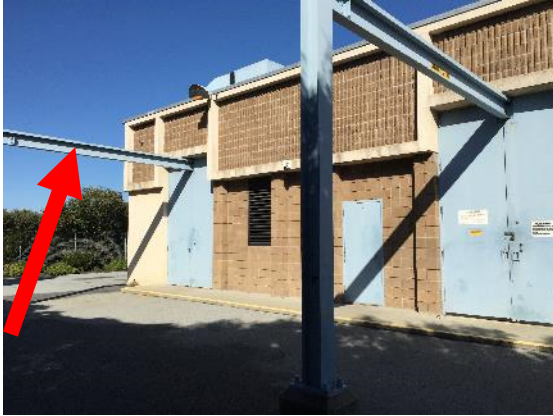
Figure 4-5 Steel Monorail at Entrances to Equipment Room (left) and to the Blower Room (right)
