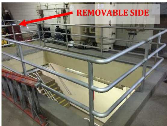
Figure 4-6 Aluminum Guardrails Around Opening on Equipment Room Floor
