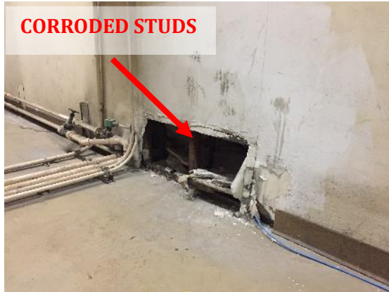
Figure 4-7 Opening in Base of Wall Between Equipment and Hyperchlorination Rooms
